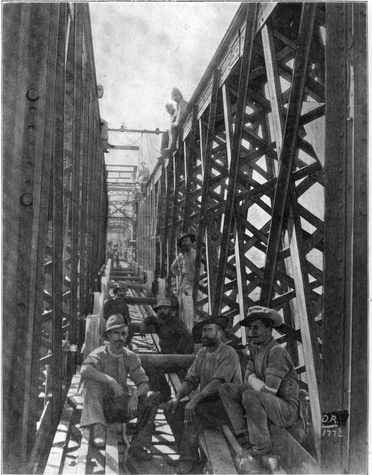
Orange River Bridge, Norval's Pont.
