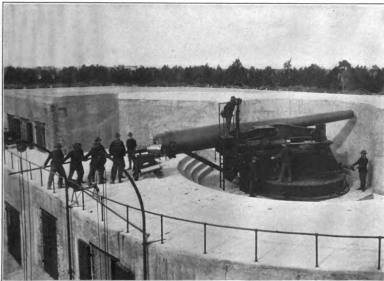
FIG. 2. Loading a Gun Mounted on a 10-inch Disappearing Carriage, Model 1896.
