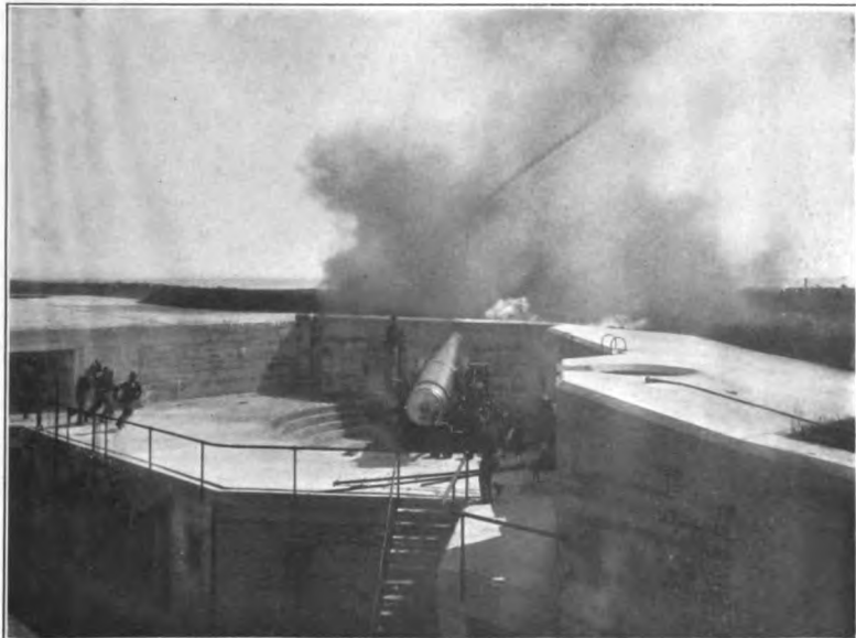
FIG. 2. Gun Mounted on 10-inch Disappearing Carriage, Model 1896. (Photograph taken about one second after firing, showing gun below the parapet.)
