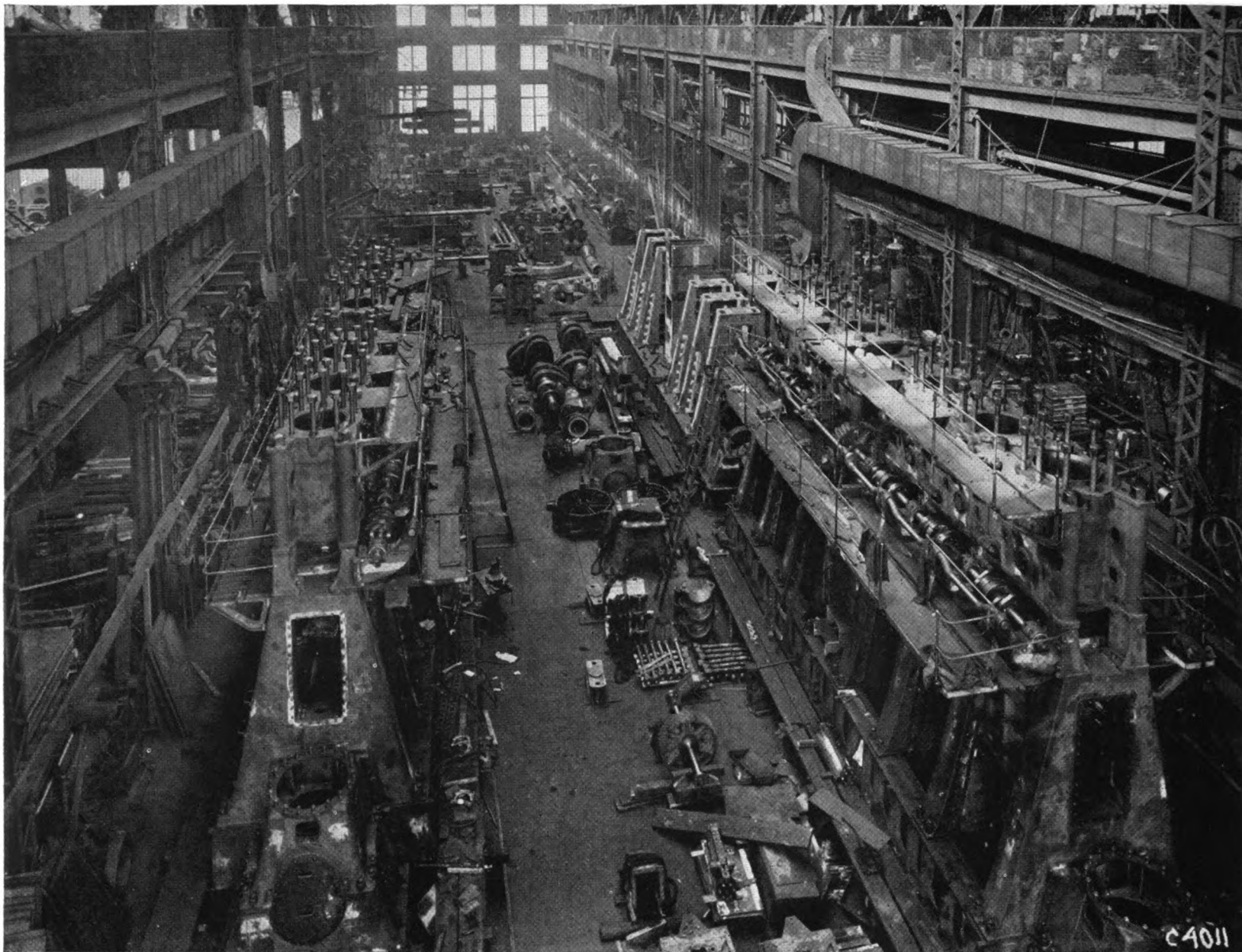
View of the main machine-and-erecting shop at the Cramp shipyard showing four 2,250 i.h.p. Diesel marine engines under construction in the foreground
