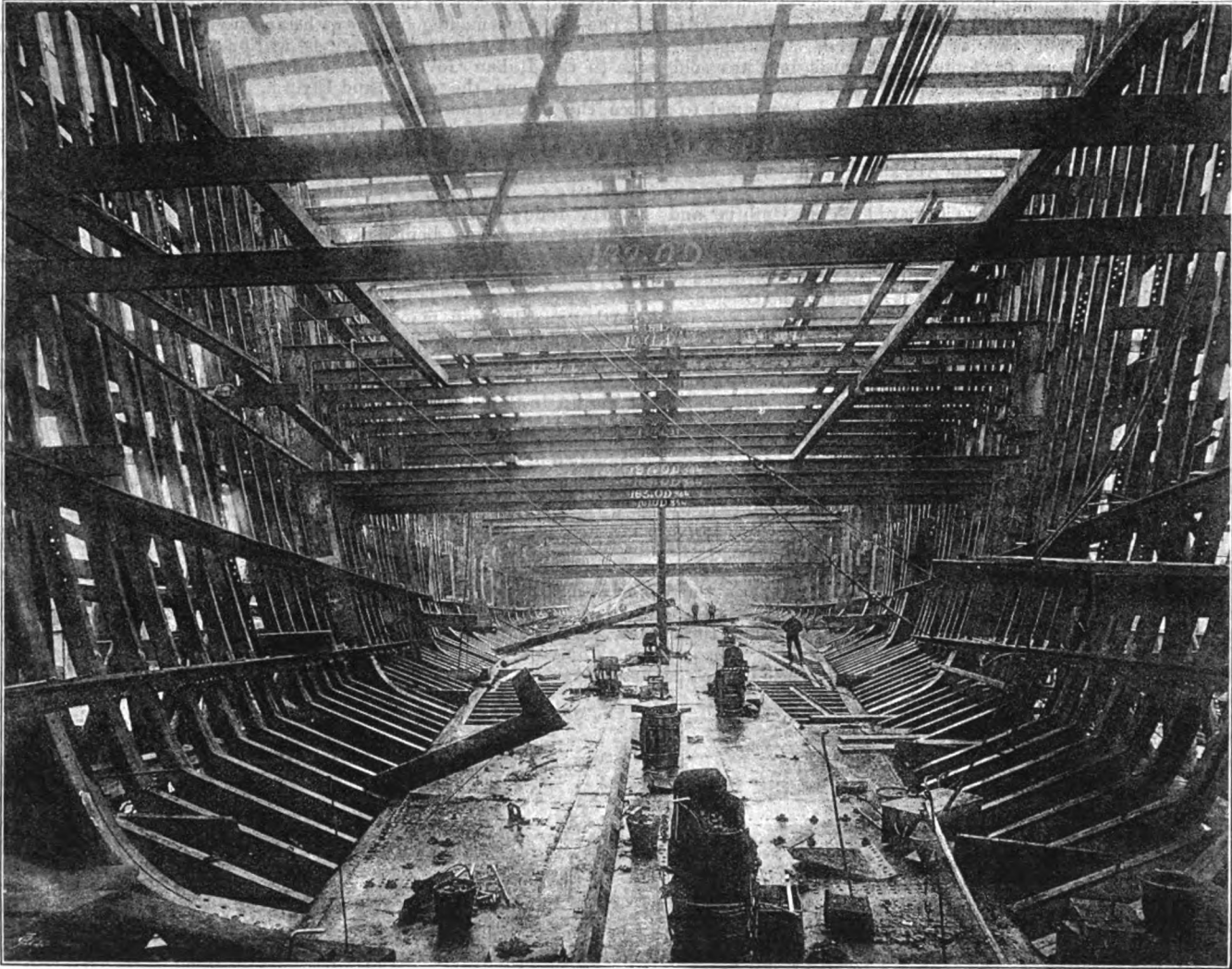
FIG. 7. MIDSHIP FRAMING, AS SEEN FROM BOW, DECEMBER 31, 1891.
