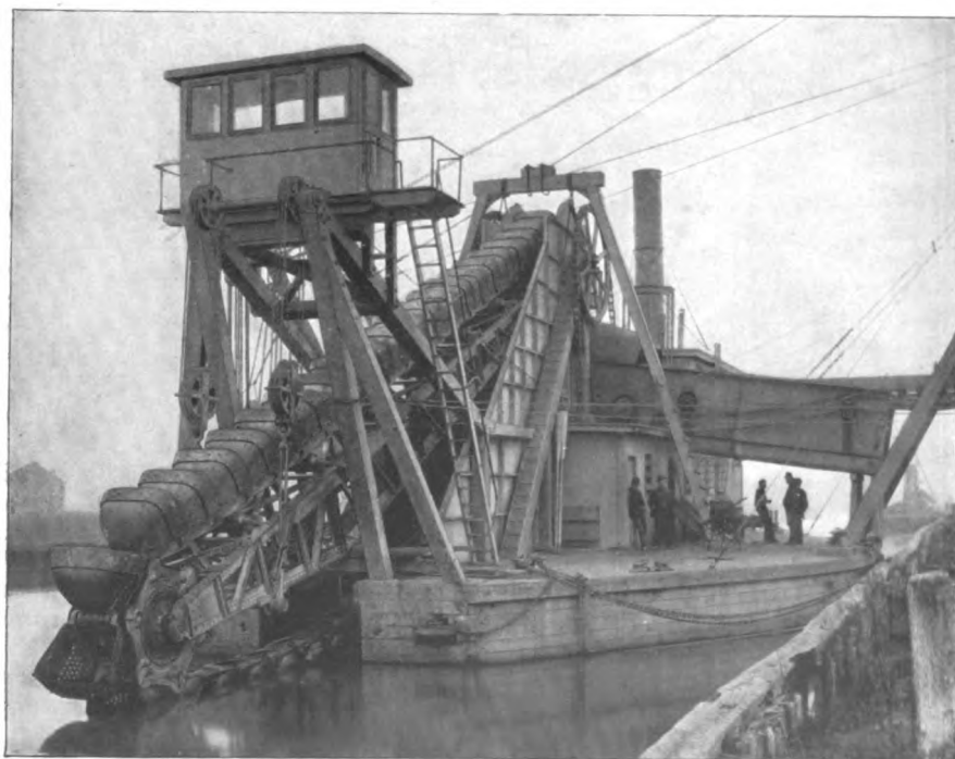
A LADDER DREDGE.
