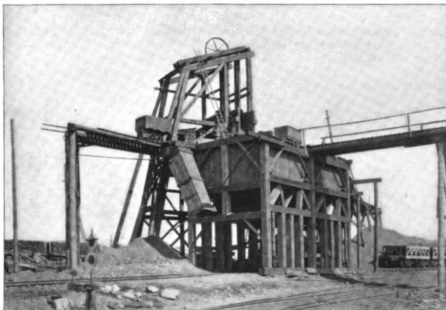
THE HEADWORKS AT A MINE.
