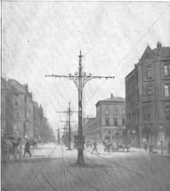
A TROLLEY LINE AT HANNOVER, GERMANY
