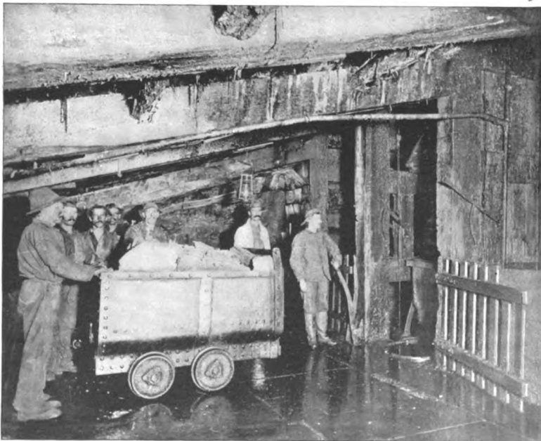
AT THE BOTTOM OF THE 4000-FOOT TAMARACK SHAFT.
