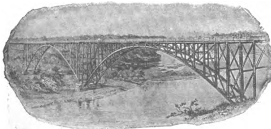
Mississippi River Bridge. Centre Spans each 456 feet.
