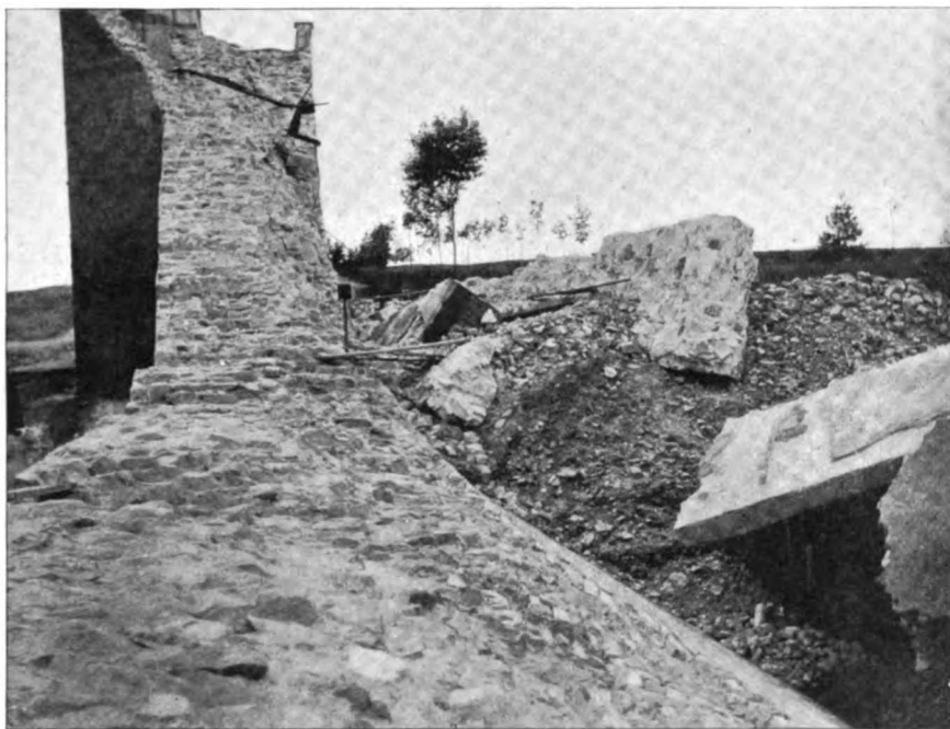
FIG. 7. LOOKING ALONG THE DAM TOWARDS THE SLUICE TOWER.
