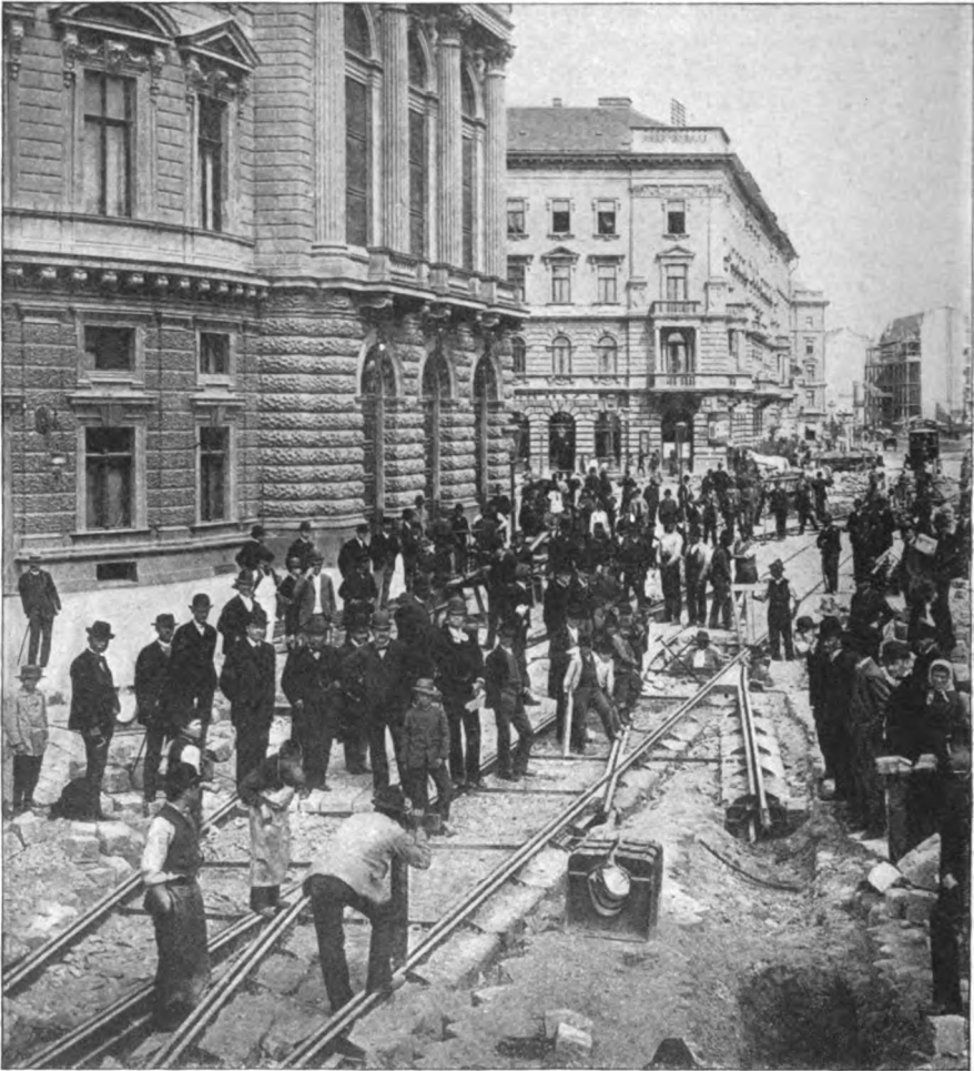
THE BUDA-PEST CONDUIT ROAD DURING CONSTRUCTION.
