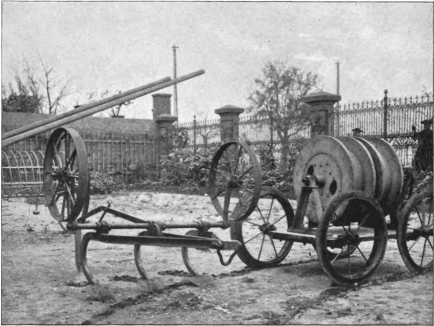
ONE OF THE ANCHORS FOR THE PLOW HAULING CHAIN.
