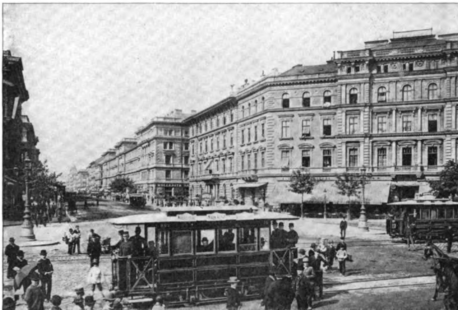
ALONG THE LINE OF THE BUDA-PEST CONDUIT ROAD, BUILT BY MESSRS. SIEMENS & HALSKE, OF BERLIN AND CHICAGO.
