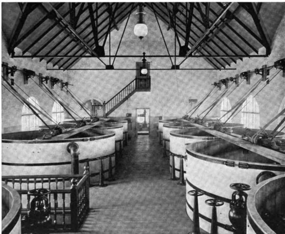
A GRAVITY FILTER PLANT AT NIAGARA FALLS, N. Y. ERECTED BY THE MORISON-JEWELL FILTRATION CO., NEW YORK.
