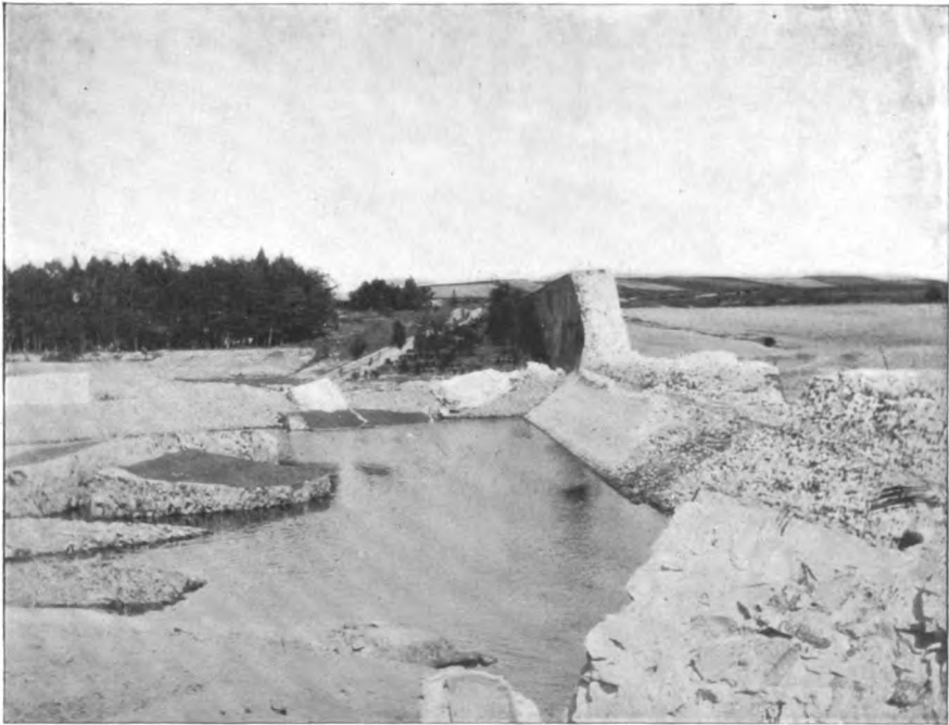
FIG. 6. BOUZEY DAM, LOOKING TOWARDS BYEWASH.
