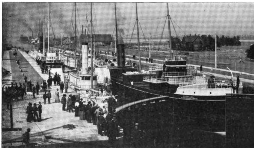
FOUR VESSELS IN THE NEW LOCK OF THE SAULT STE. MARIE CANAL, GIVING A GOOD IDEA OF ITS SIZE. LENGTH, 800 FEET. WIDTH, 100 FEET.
